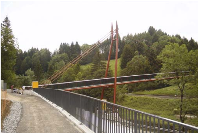
Fig. 15 Side view of Bennaer Steg
